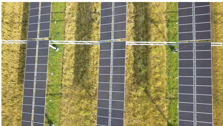
The agrivoltaics pilot plant by Fraunhofer Institute for Solar Energy Systems at the Heggelbach farming community in the south of Germany. Solar modules are mounted 5 to 8 meters above ground with supports spaced in ways that allow the operation of normal farm machines. Credit: Tobi Kellner via Wikimedia Commons
